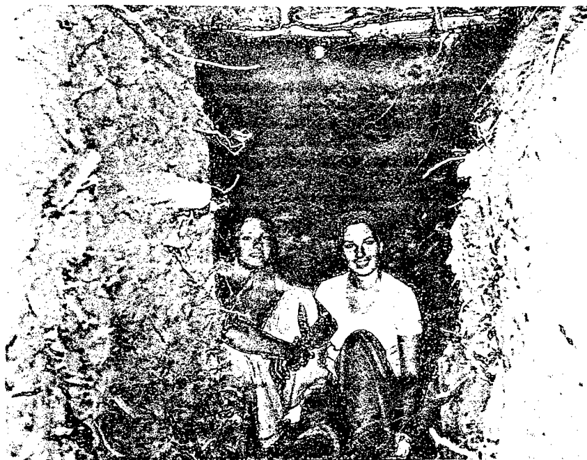
Fig. 5.2. Two non-athletic college girls who completed a 4-person Pole-Covered Trench Shelter in 35\frac{1}{2} hours, despite tree roots.
