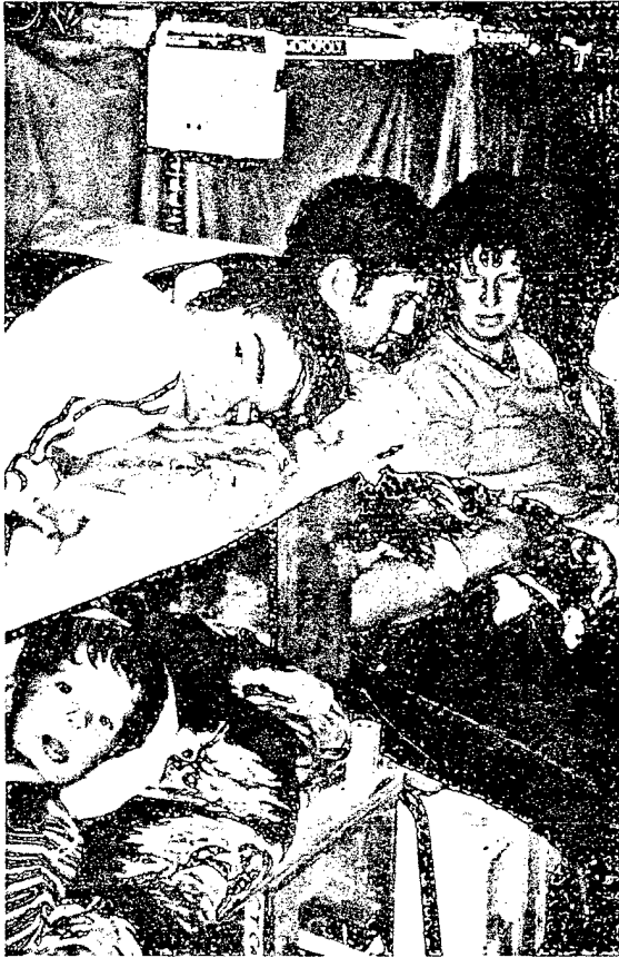
Fig. 14.1. Bunks and folding chairs furnished this Pole-Covered Trench Shelter. (Note the suspended transistor radio. Reception is good in all types of expedient shelters tested to date.)
