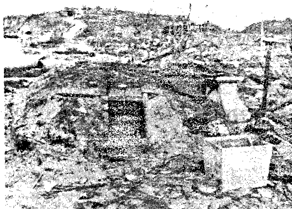
Fig. 1.5. Undamaged earth-covered family shelter in Nagasaki.
