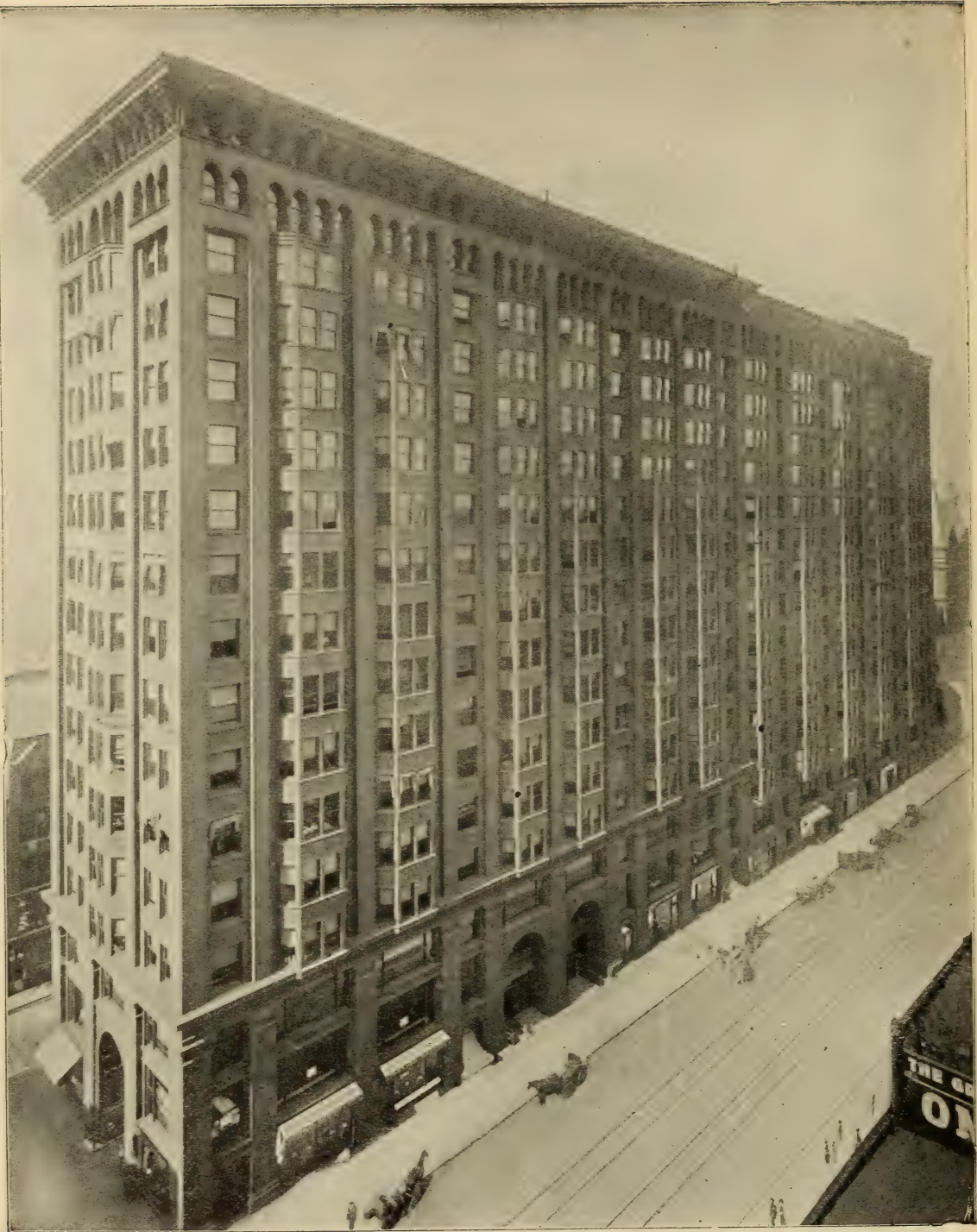
MONADNOCK BUILDING, CHICAGO, ILL.
