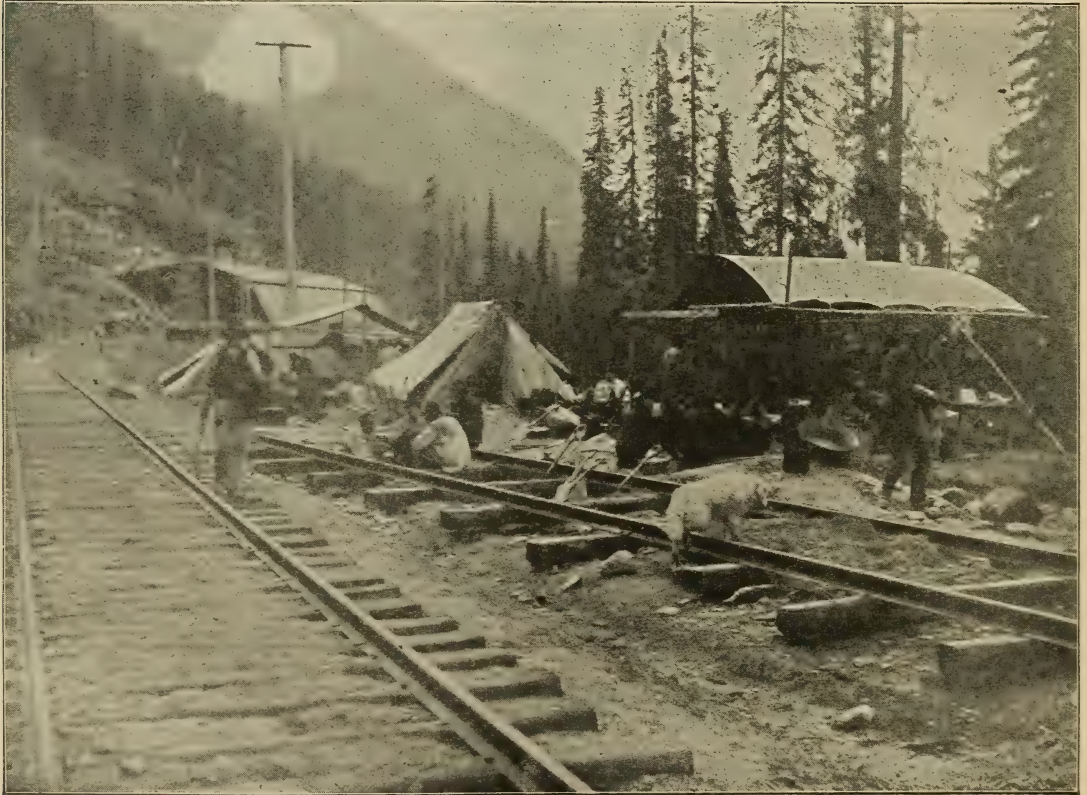
RAILWAY CONSTRUCTION IN THE MOUNTAINS.
