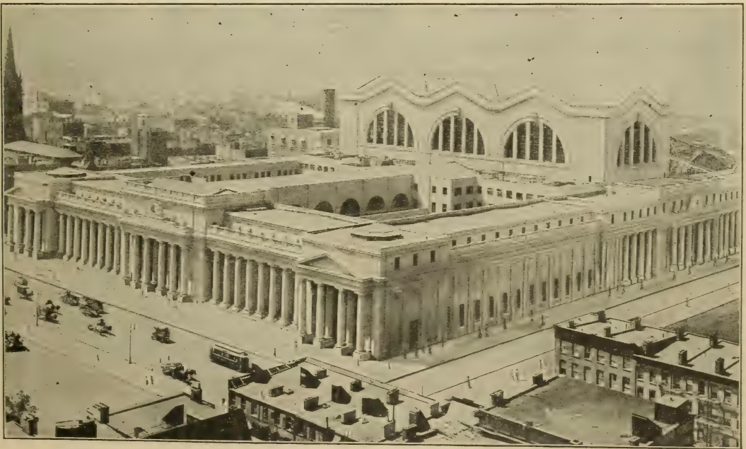
MONSTER NEW STATION OF PENNSYLVANIA RAILWAY IN NEW YORK. This picture shows only one-third of length of structure.
