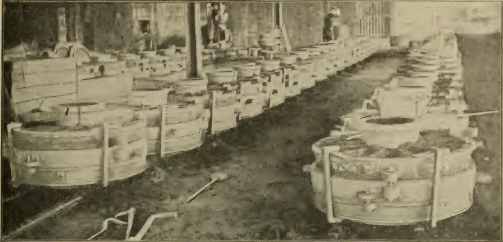
MAKING CAR WHEELS—MOLDS READY FOR POURING.
