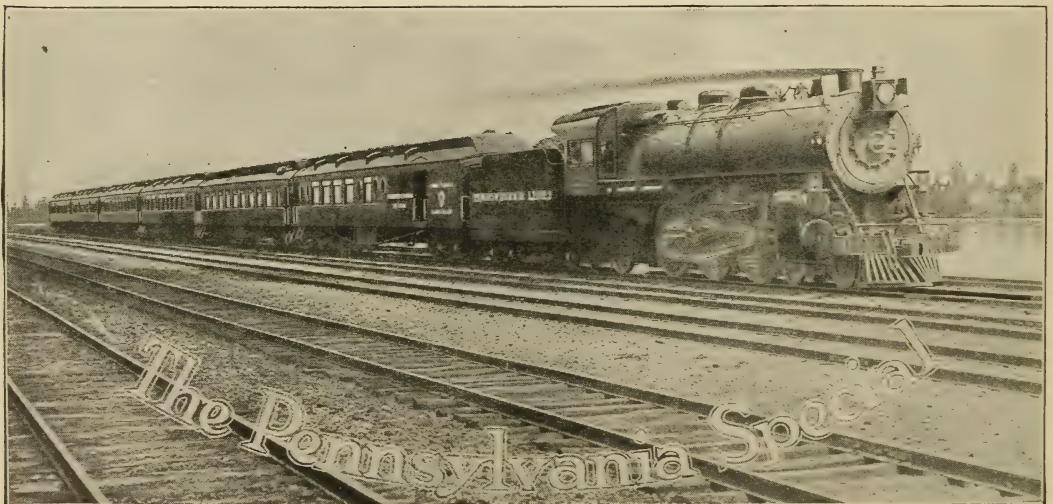
FIRST ALL-STEEL CAR TRAIN IN OPERATION. The newest invention in railroading—will not break to pieces and cannot take fire.
