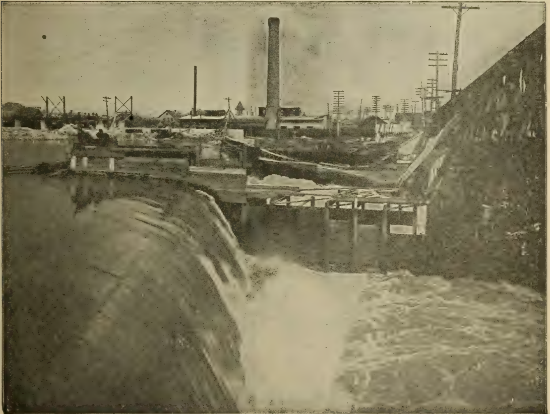
DAM AT LOCKPORT, ON THE CHICAGO DRAINAGE CANAL.
