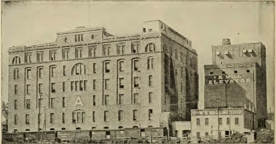
PILLSBURY "A" MILL. THE LARGEST FLOUR MILL IN THE WORLD. CAPACITY, 15,000 BARRELS DAILY.
